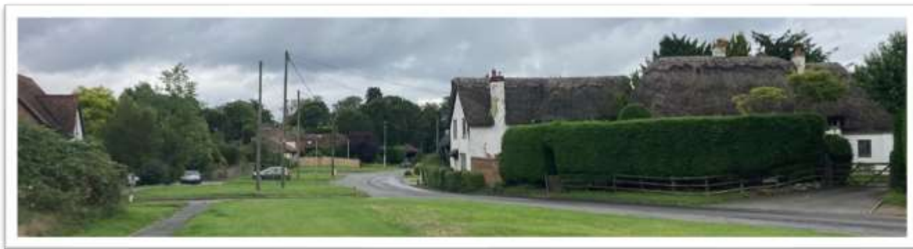
Drayton Road looking towards the Newton Longville Conservation Area
