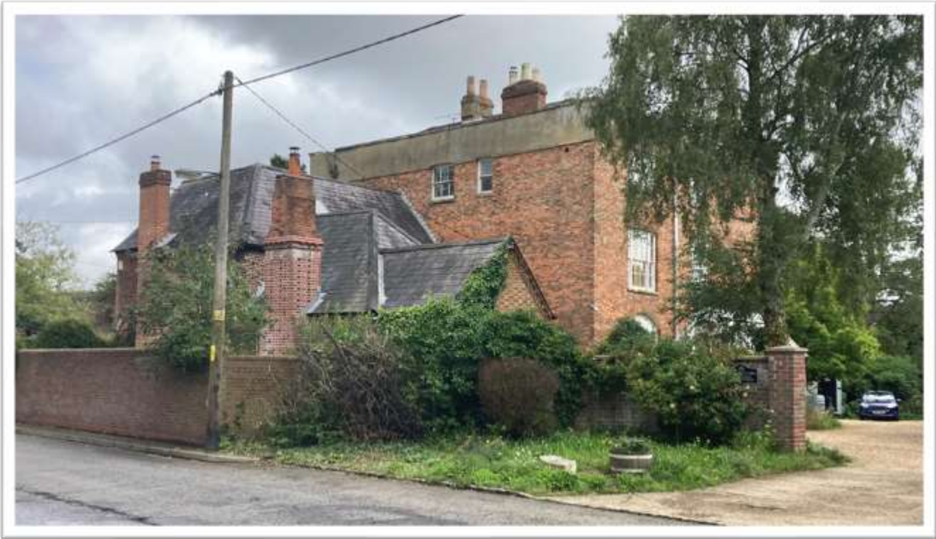
The Grade II listed Flat, the Old Parsonage and the Old Rectory, Drayton Road
