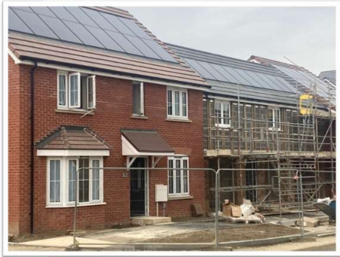
New build with roof solar panels
