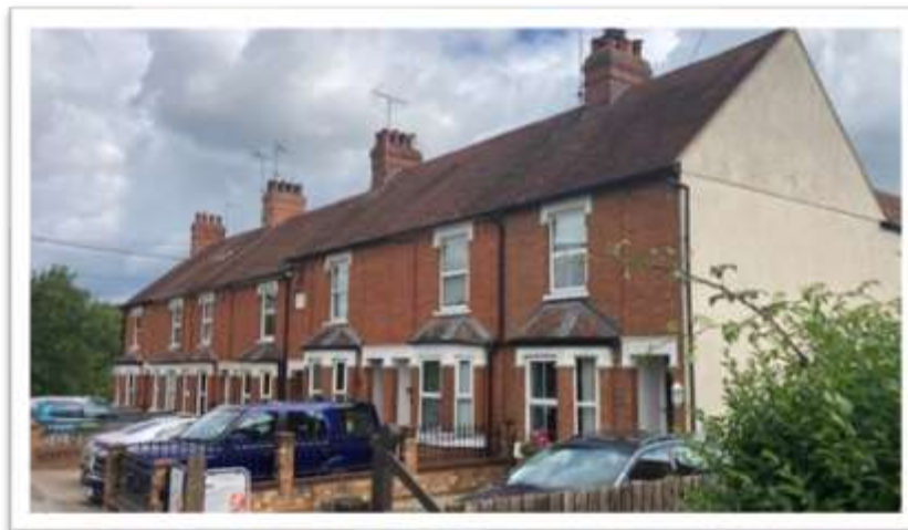
Brickworks cottages, 108-120 Bletchley Road
