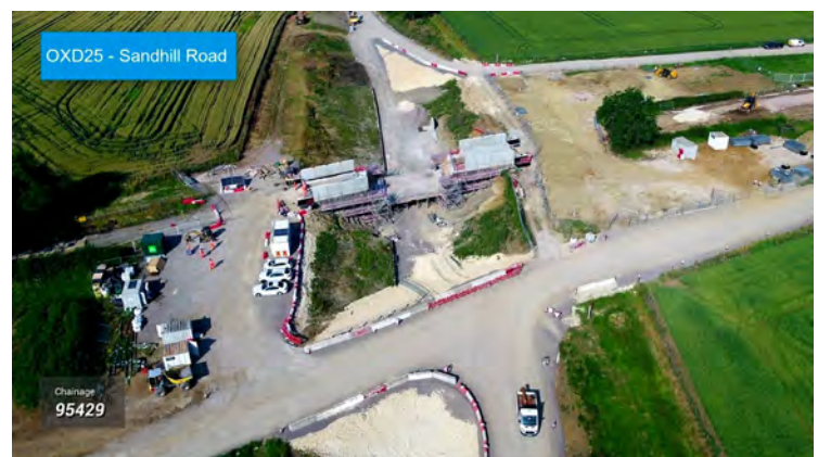
Sandhill Road overbridge from above (taken Mid July 2021)
