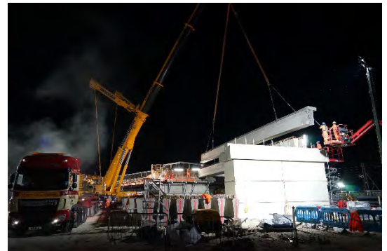
A beam is lifted into place on Bletchley Flyover
