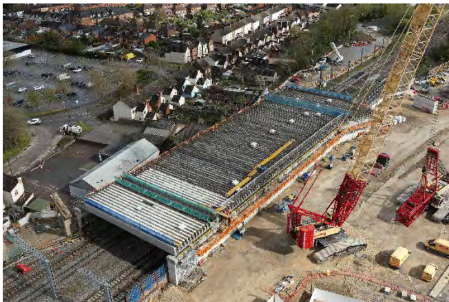
103 precast concrete beams were lifted into place over the West Coast Main Line
