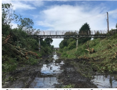
Site clearance in the Winslow Cutting
